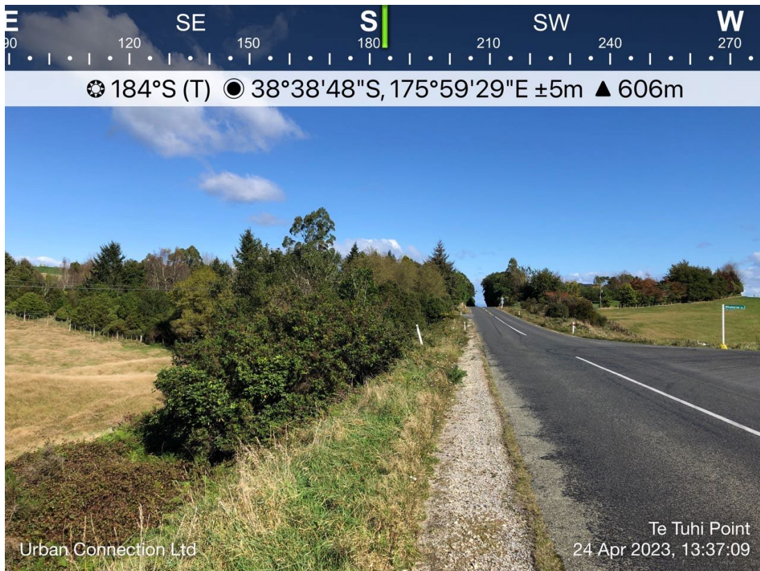
Figure 6: Steep bank opposite Whakaroa Road and Mapara Road intersection
