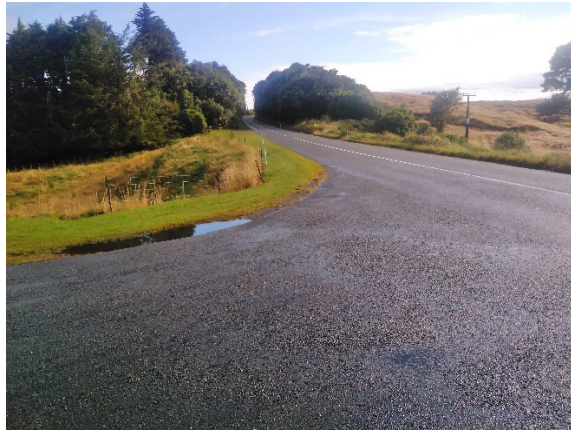
Figure 18: Sight distance from the Whakaroa Road and Mapara Road intersection to the North
