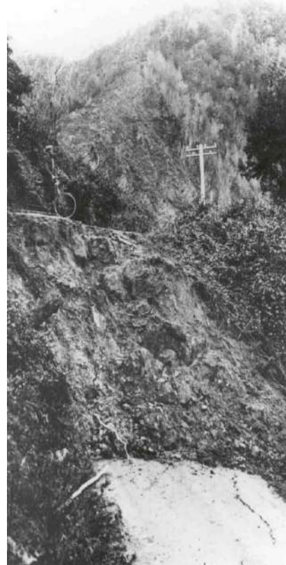
b) White Creek Fault – The 1929 Murchison earthquake resulted in over 4 m of vertical displacement of the ground surface at the White Creek fault (Berryman 1980). Note the cyclist standing on the upthrown side of road that is displaced by the fault.
