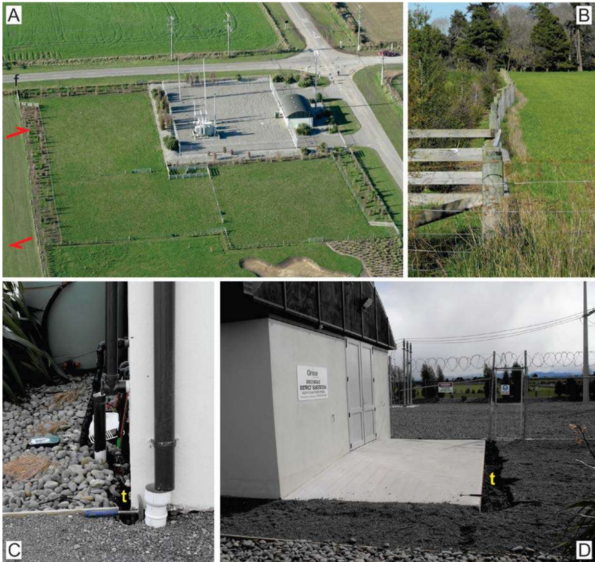
Figure A2.12 Greendale substation and Greendale Fault surface rupture; see Figures A2.7 and A2.8 for location. (A) Aerial view looking northeast. Red arrows denote location, strike and sense of lateral displacement of the surface rupture deformation zone. Photo by Richard Jongens. (B) View looking southwest along fence line adjacent to the substation that crosses the surface rupture deformation zone and records the amount, width and distributed style of fault displacement here (camera location for B is shown by black 'f' in (A)). Photo by Russ Van Dissen. (C, D) Views looking northwest. 't' is where soil has pulled away from the building's foundation. See text for details. Photos by Russ Van Dissen.
