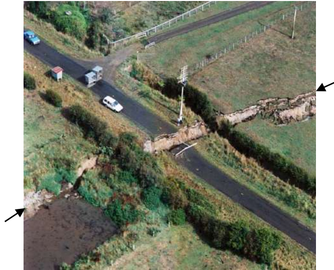
a) Edgecumbe Fault – The 1987 Edgecumbe earthquake resulted in about 7 km of surface rupture along the Edgecumbe fault, and up to about 2 m of vertical displacement of the ground surface at the fault (Beanland et al 1989). Arrows mark the location of surface fault rupture.
