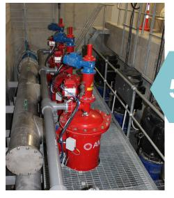
The black and blue water pumps (on the right) take the raw water from the lake through the strainers and membranes into the treated water tank. The red strainers protect the membranes from any debris by filtering out any material larger than 0.3 mm.
