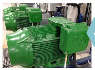
These three green water pumps move the treated water to Tamatea and Titoki reservoirs.
