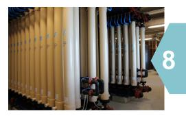
The filtration membranes remove any remaining particles larger than 0.1 microns. A micron is one thousandth of a millimetre – so a particle has to be miniscule to get through this process.
