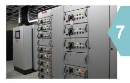
The Motor Control Centre houses all the electrical equipment that operates the plant including the controls that alter the speed of the motors and pumps.
