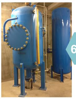
The large blue tank is full of compressed air, which is used to keep parts clean, provide a cushion in the surge vessel and operate various valves.
