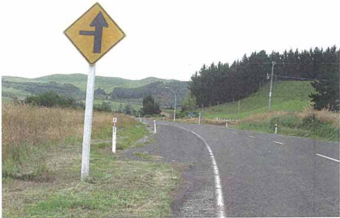
PHOTO 5 – SH32 NORTH APPROACH TO KURATAU HYDRO ROAD NOTE: PW-11 SIGN IS 170M FROM INTERSECTION
