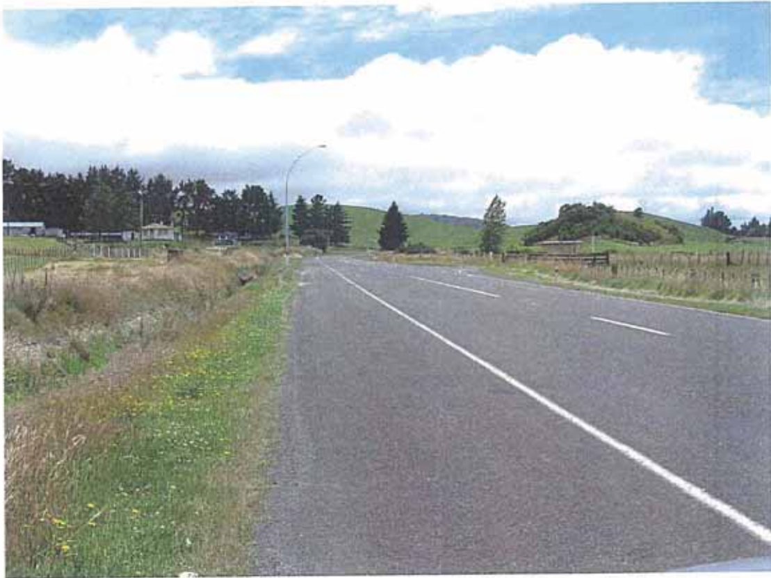
PHOTO 1 – SH32 SOUTH APPROACH TO KURATAU HYDRO ROAD NOTE: INTERSECTION SIGNS
