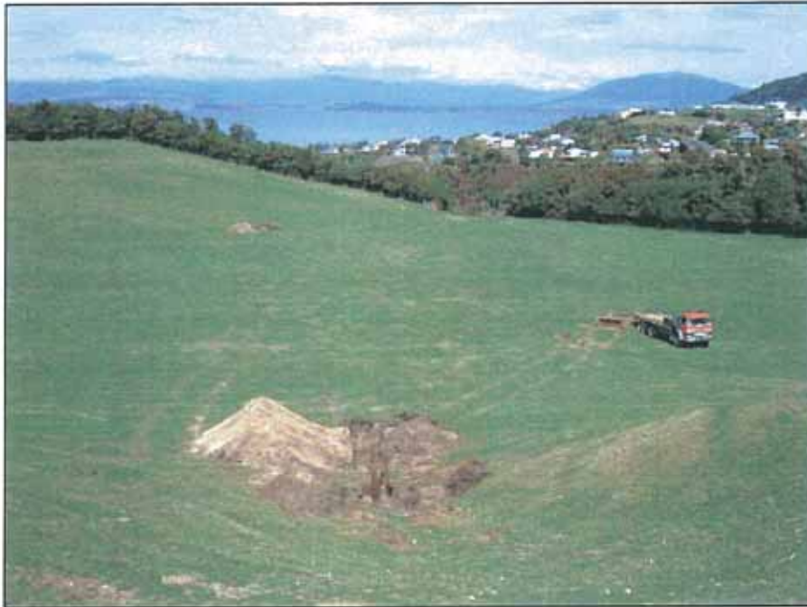
Fig. 1: View south towards the low-lying area with Lake Taupo in the distance. Test Pit No. 1 is in the foreground.
