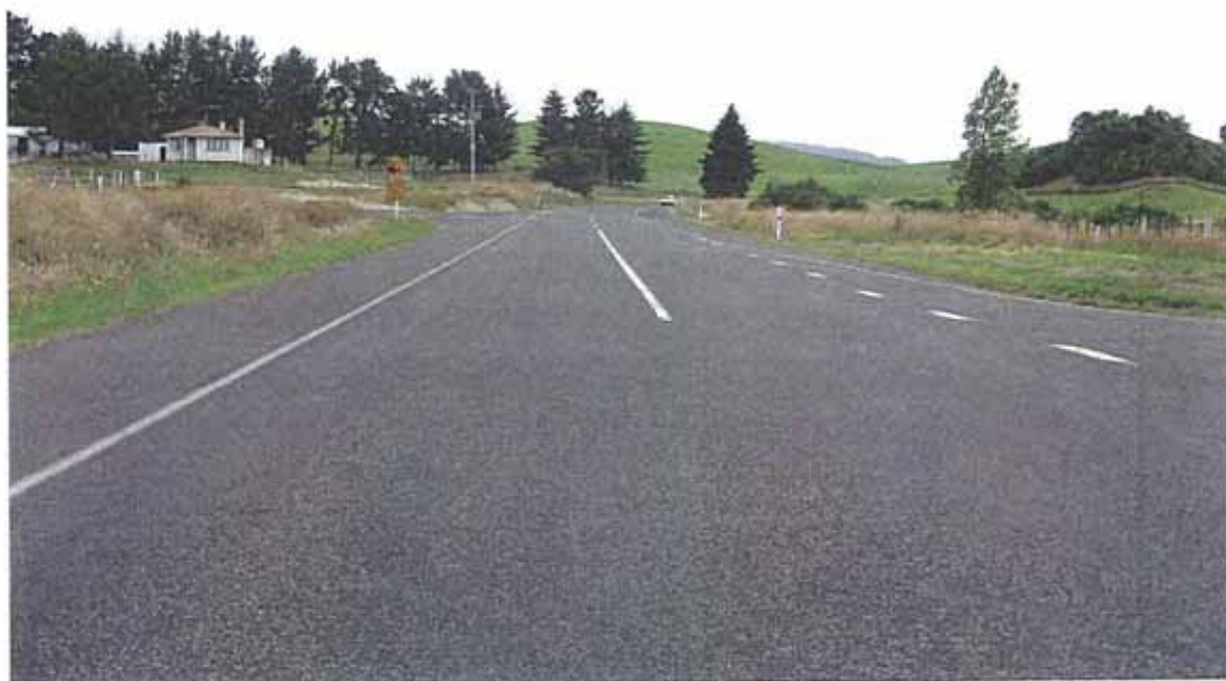
PHOTO 4 – LOOKING NORTH ALONG CENTRELINE OF SH32 FROM INTERSECTION NOTE: PW-11 “SIDE ROAD CONTROLLED” SIGN BESIDE VEHICLE
