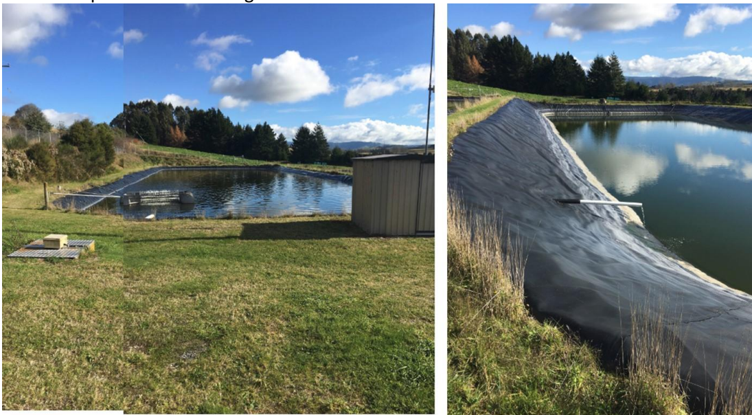
Figure 3: Whareroa Wastewater Treatment Plant (Pond 1 at left, Pond 2 at right)
