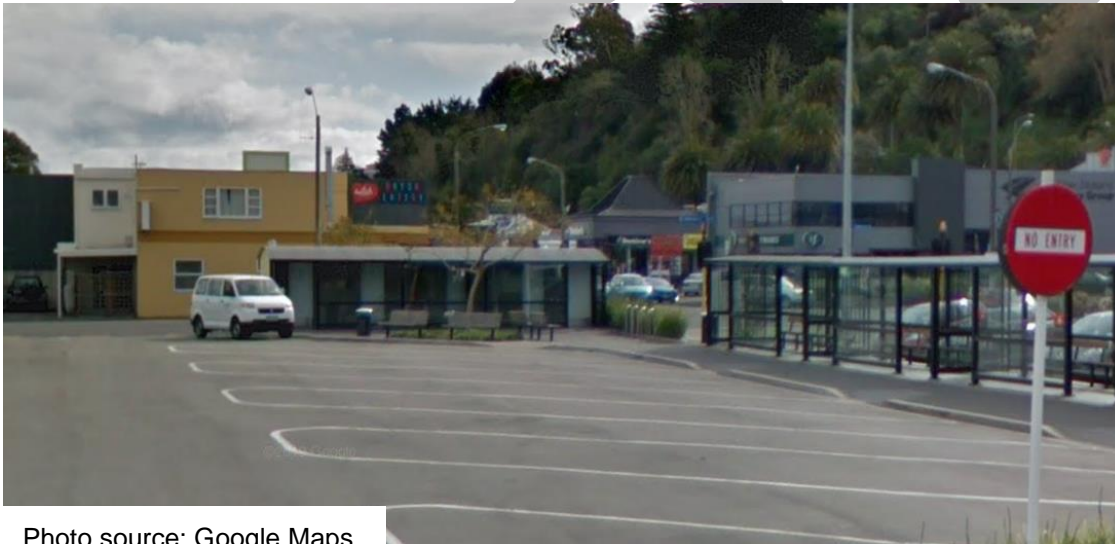
Napier offstreet bushub, with bus angle parks, public toilets and glass shelters
