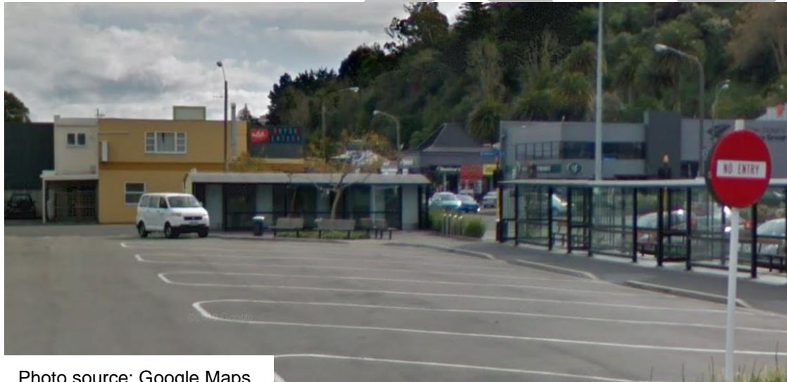
Napier offstreet bushub, with bus angle parks, public toilets and glass shelters
