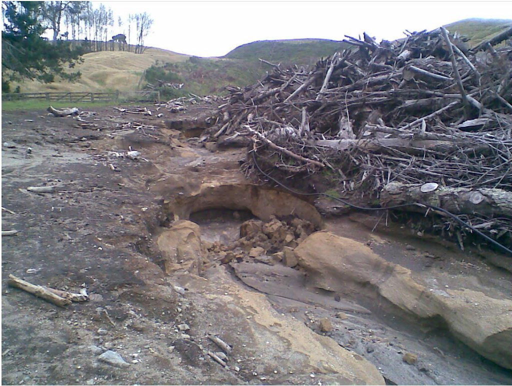
Upper Nukuhau erosion caused by stormwater within a gully system with no vegetative protection, 2012.
