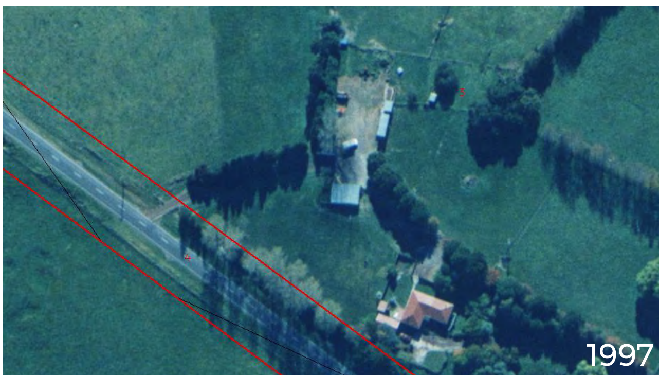
2007 to 2016 – Some storage sheds have been removed. Residential property has been demolished and foundations are visible.
