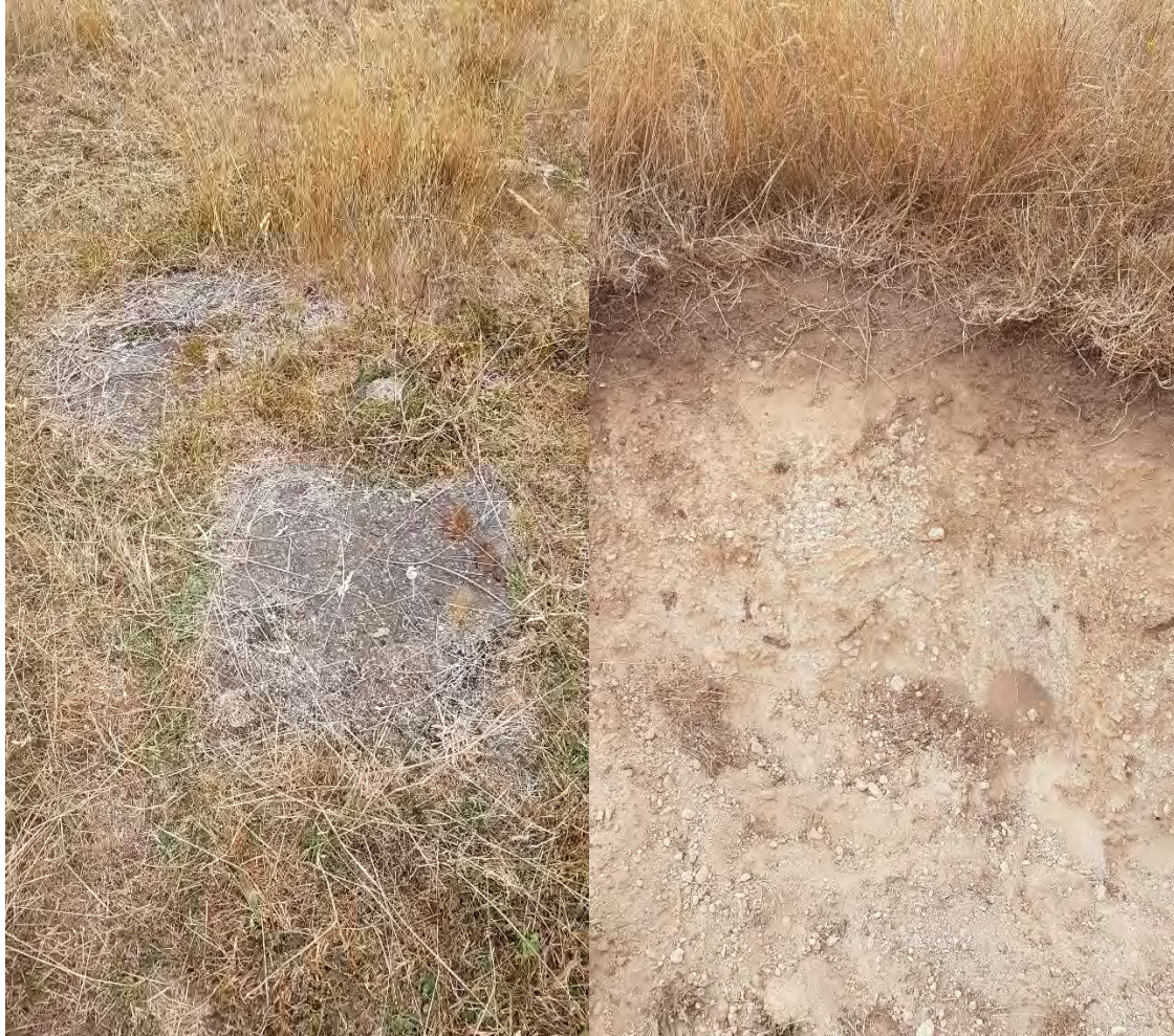
Concrete footings (left) and exposed natural ground (right)
