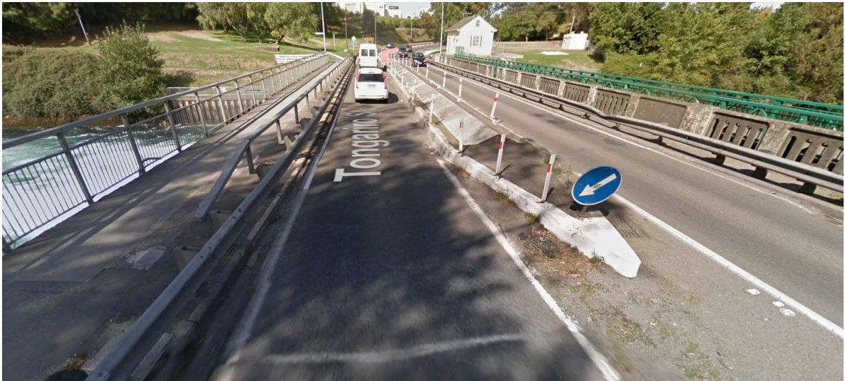
Figure 2-4 Control Gate Bridge Looking South
