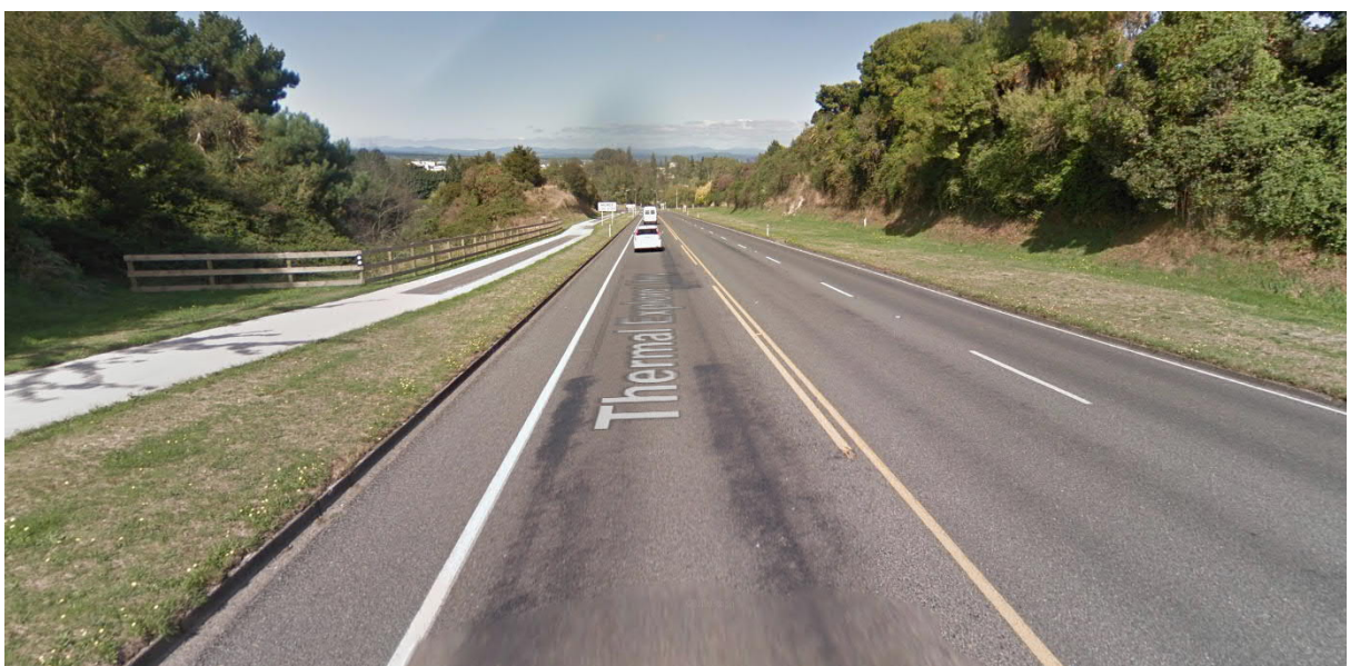
Figure 2-3 Wairakei Drive Approaching Control Gate Bridge Looking South
