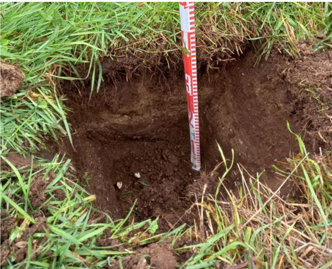
Figure 15: Test pit dug within Figure 9 depression.
