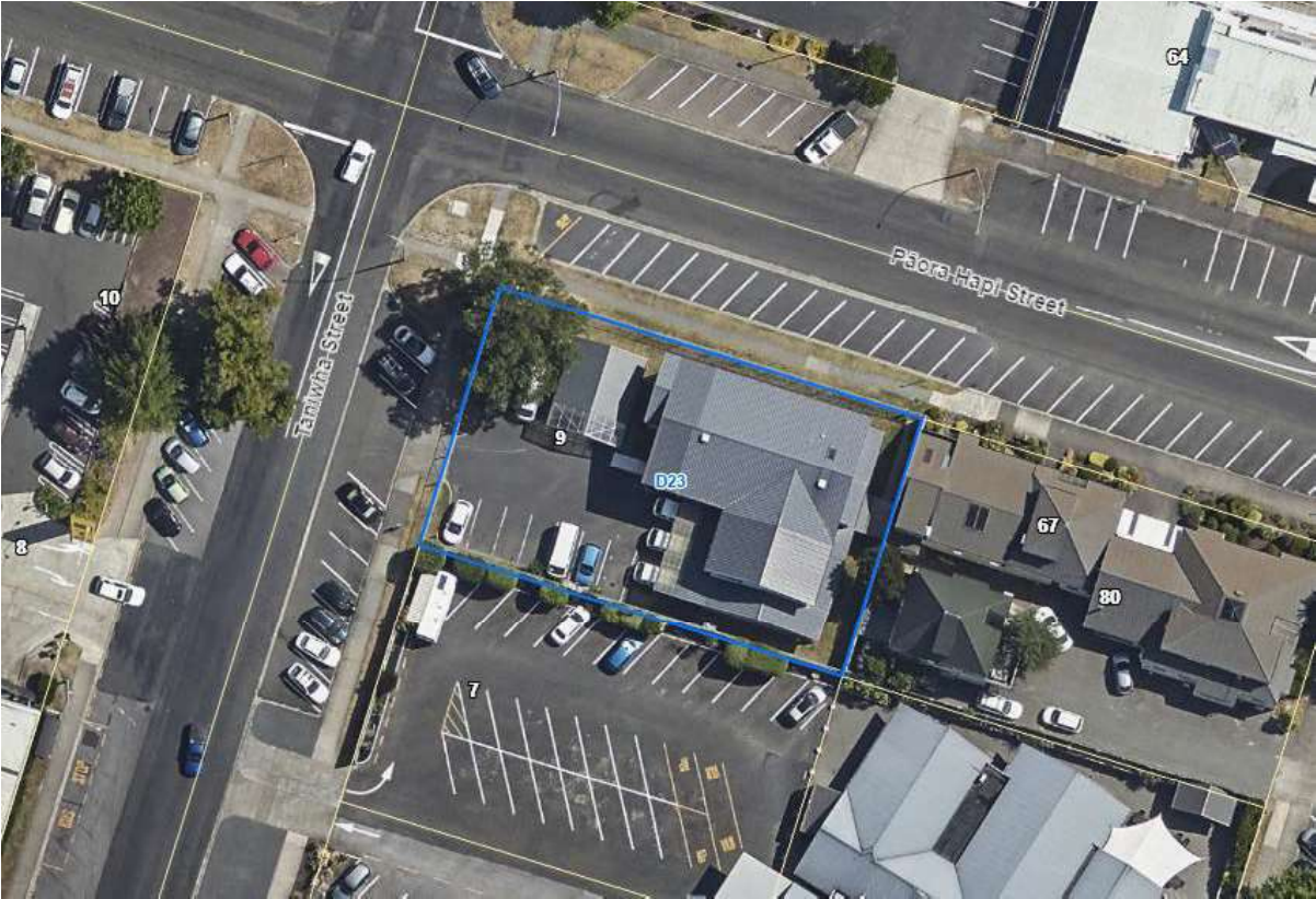
Figure 3: Aerial photograph of the Taupō Community Corrections site ('D23') Source: Taupō District Council GIS
