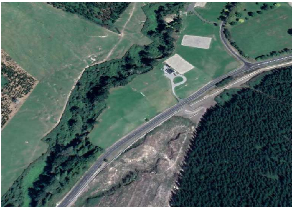
Figure 1 Section of Poihipi Road with a geothermal pipeline running alongside the road (right hand side)
