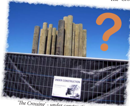
"The Crossing" - under construction
